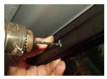
Using the compression frame's predrilled holes as a guide, start drilling pilot holes in the middle of the window with an 1/8-inch bit. Mount some screws lightly, and continue around the perimeter of the window until all the holes are drilled and screws mounted. Be careful to drill the holes on the bottom of the window near the bottom of the frame. The screws must go beneath the window screen's track.
